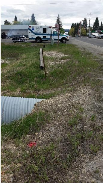
Some additional material is need to adjust slope in this section. This begins 340' of asphalt.
