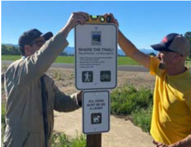
Wes Keller, left, and Tyler Busby help install the trail signs for the Heinrich Demo Trail. Thanks guys!
