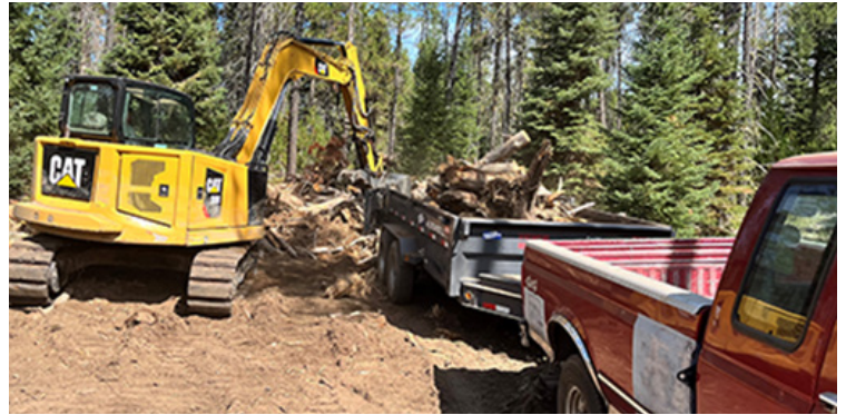
Josh Murrey, operating the excavator, places dead wood into a dump trailer pulled by Steve Stuebner's pickup truck. Thanks to Tom Mihlfeith and Eric Gehrung for donating their time, p/u trucks and dump trailers for that effort, too.
